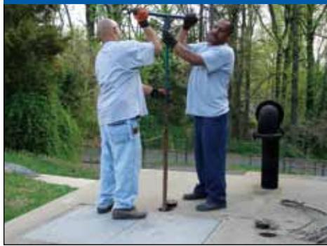
Crew members close a valve at a water pumping station. Closing the upstream and downstream valves on a segment of water main will stop the flow to a broken section.
