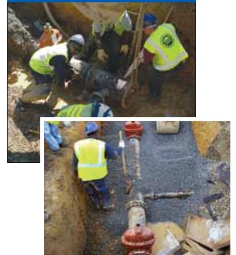
A new segment of pipe is positioned in place. Once connected, the water main is returned to service. After ensuring the main has been repaired satisfactorily, the trench is backfilled. Proper backfill and compaction reduce roadway settling.
