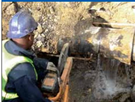
A cracked section of pipe is removed. In this case, a 12-inch pipe at Kirkwood Rd. and Washington Blvd. split at the joint and needed to be replaced.
