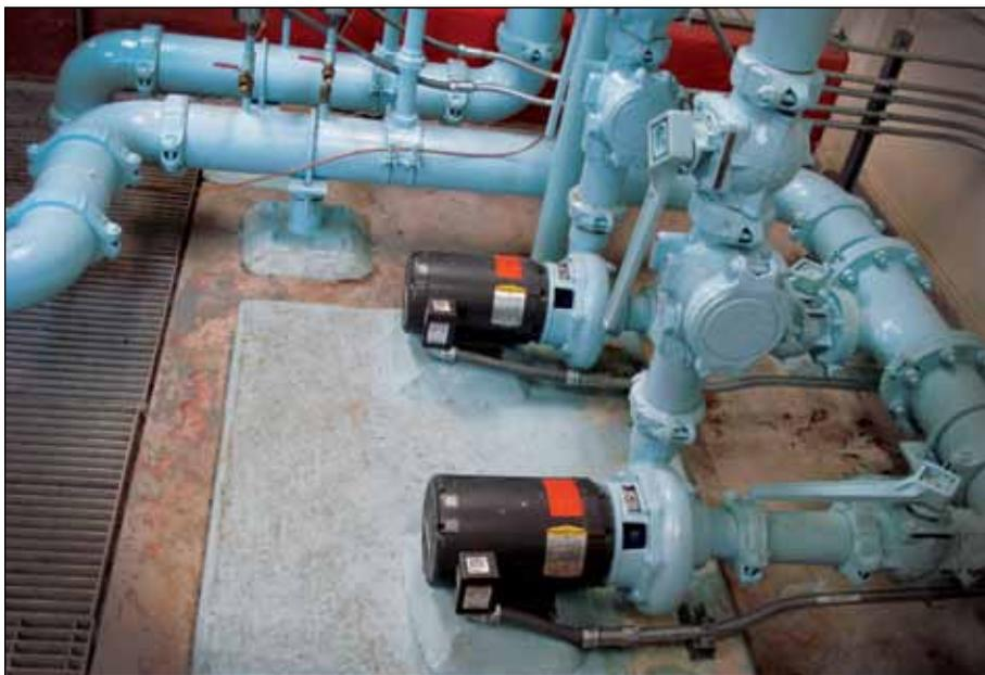
Installed in 2009, these booster pumps at Arlington's Minor Hill facility provide improved water pressure to the surrounding area.
