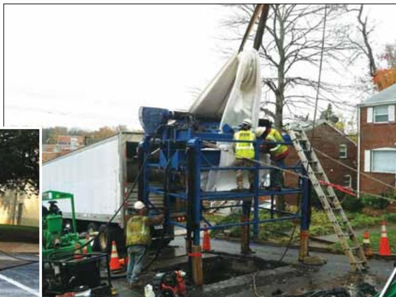
The most common method of rehabilitation of sewers is done using CIPP, a process in which a resin-impregnated felt liner is pushed into the existing pipe to make it stronger and better sealed. CIPP reduces sewer flows to the Water Pollution Control Plant by preventing groundwater from entering the pipes.
