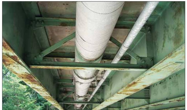
This 12-inch water main under the S. Abingdon Bridge crossing Interstate 395 is the first water main in Arlington that was rehabilitated using the cured-in-place pipe technology.
